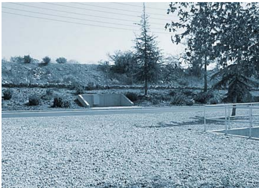
Pictured Above: Probable location of storage basin connection at Miramar.
